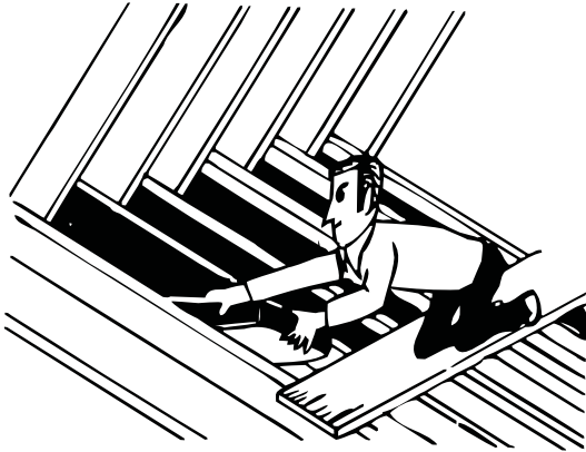
Laying batts in the attic with vapor barrier down.
