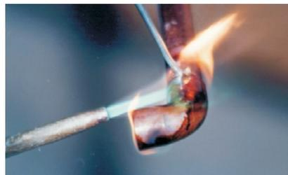
Touch the solder to the pipe/tubing where it joins the fitting. The heating action will pull the molten solder into the joint.
