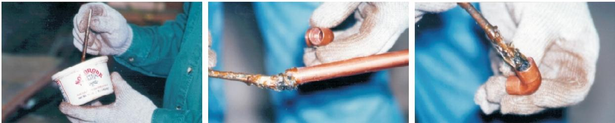
Apply flux to the outside of the pipe/tubing and inside of the fitting.
