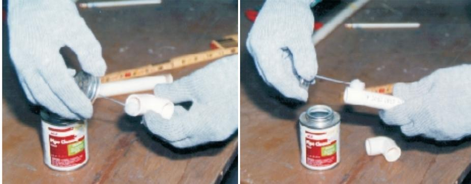
Use PVC cleaner inside the fitting and outside the pipe.
