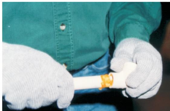
Insert the pipe into the fitting snugly and make a  $\frac{1}{4}$  turn.
