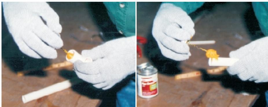
Coat the inside of the fitting and outside of the pipe with cement.
